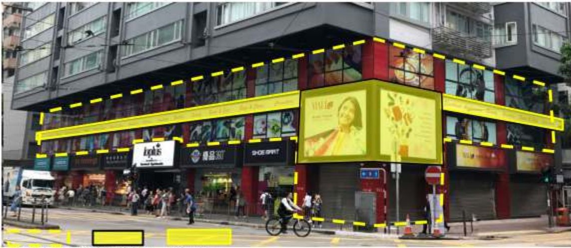
The Premises Signage Position Light Boxes
